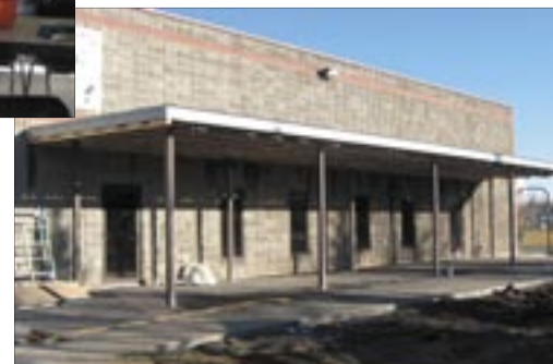
Pict 2: Oct 2010 - New Windows and Doors are installed with patio area is still under construction.
